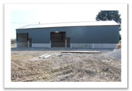
This is the front view showing where the doors are to be fitted. There is quite a large area in front of the building which will be levelled and covered in tar planings. There will also be a security fence on the right hand side.
