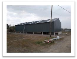
April has seen a lot of progress as many of you will have seen on Face Book. The whole structure is now complete with sides, roof and windows. Next to come are the concrete floor and land drains followed by the two roller doors.
